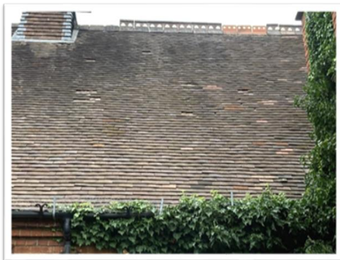
Photo 1: Ridges tiles are broken or have been replaced with a poor match. (Original ridge tiles centre)
