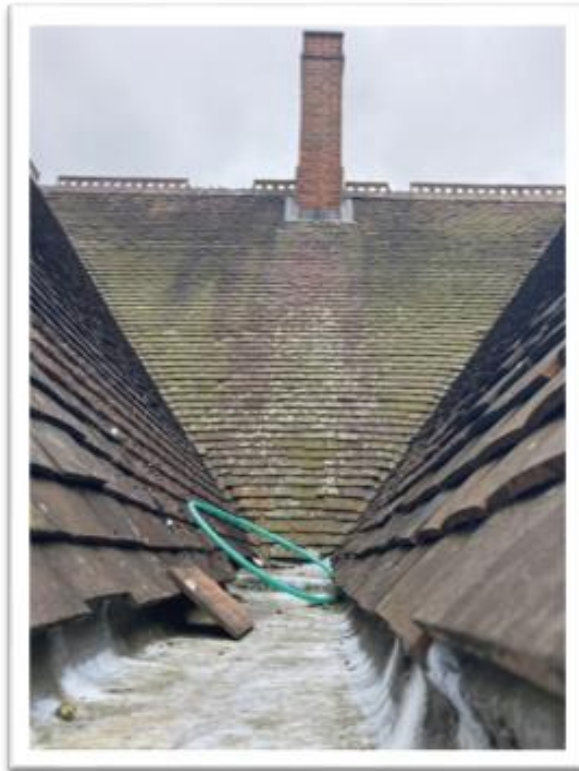
Photo 2: Typical lead gutter between roofs (Also show further tile & ridge damage)
