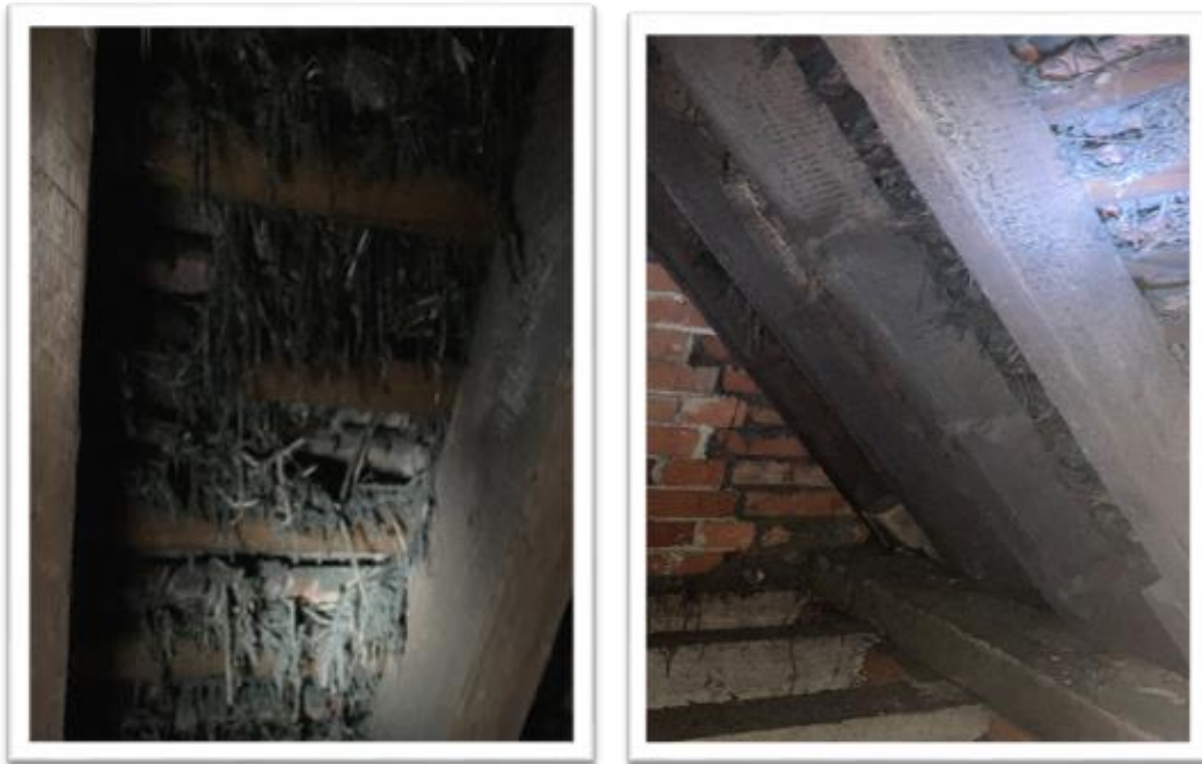
Photo 5 & 6: Remains of possible straw and plaster torching below tiles where roof voids accessible.
